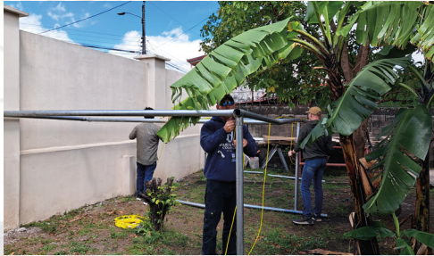
Above: Constructing the framework for the sanctuary wall boards.
